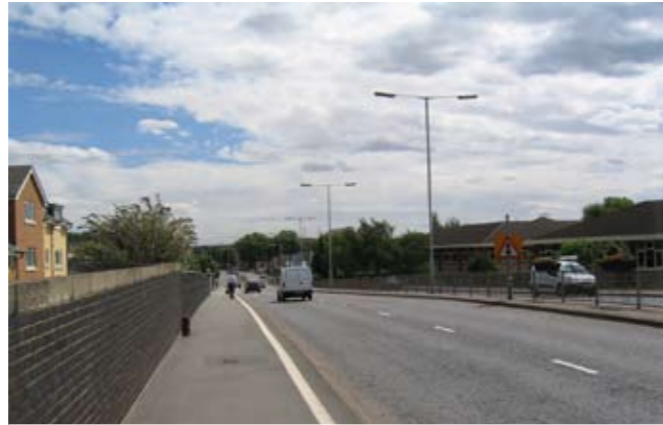
ROADWAY BRIDGE OVER RAIL LINE (ELEANOR CROSS RD)
