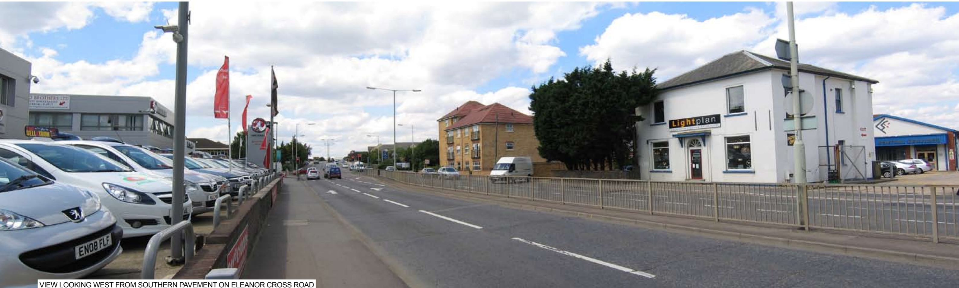
VIEW LOOKING WEST FROM SOUTHERN PAVEMENT ON ELEANOR CROSS ROAD
