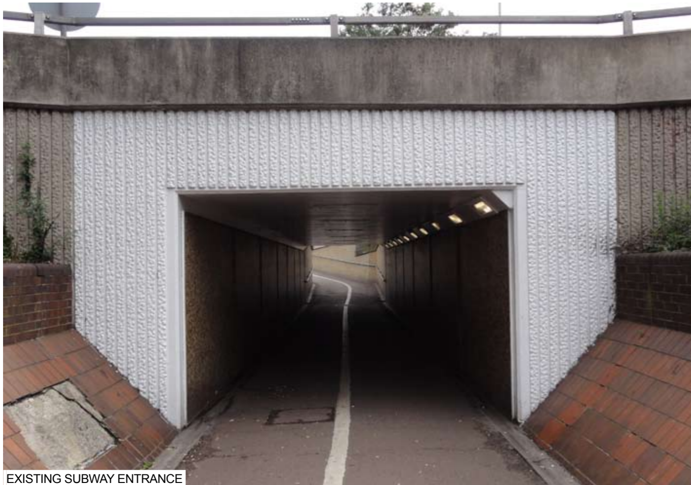
EXISTING SUBWAY ENTRANCE
