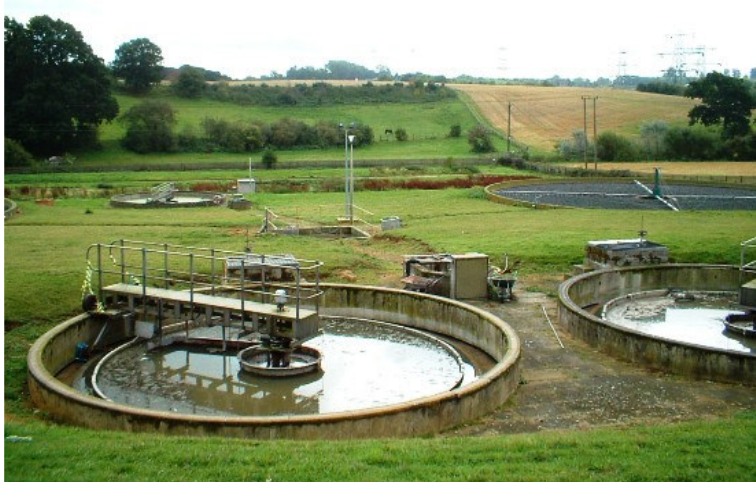
Figure 7-35 Existing settlement tank at Ashbrook WwTW
