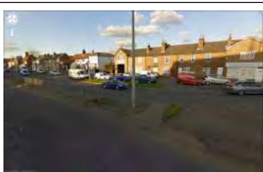
Plate 3 – eastbound view across Amwell Street showing existing informal crossing facility
