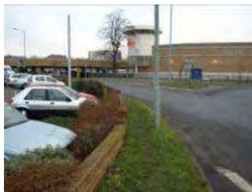
Plate 2 – lack of footway on the western side of Charlton Way past Netto car park
