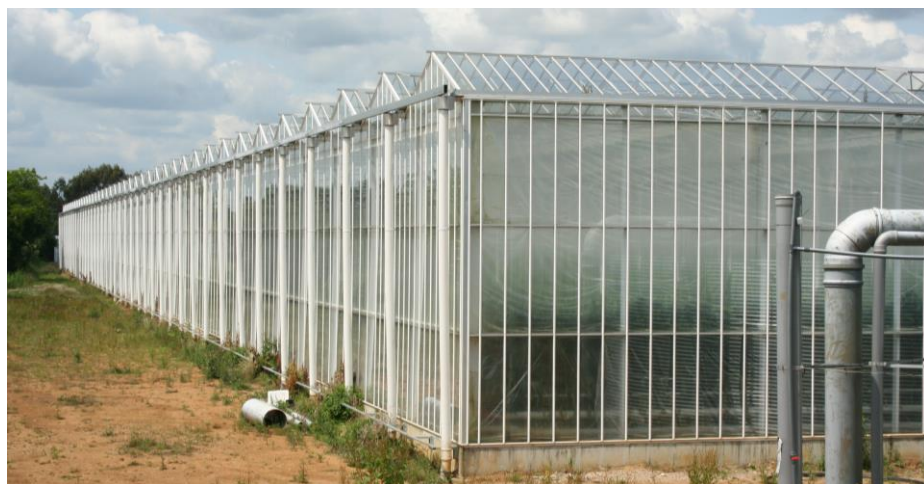
Modern 6 metre eaves glasshouses, located in Roydon in Essex
