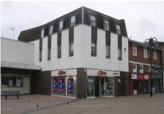
Fig 34. 'Clinton Cards'; corner building, west side of High Street.
