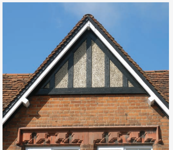
Former Three Cups Coffee Tavern, detail of gable and lintel
