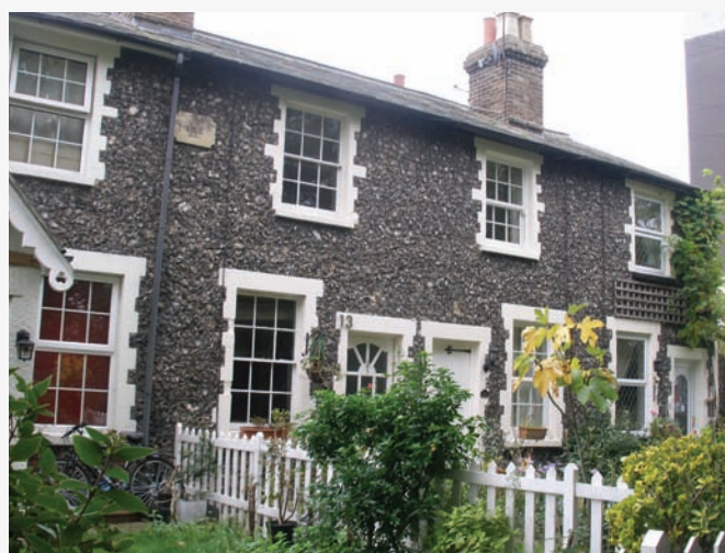
Burford Place: detail showing the contrast of the flints and painted stone dressings.
