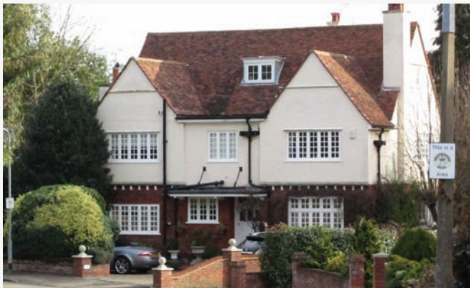
Little Whit Hern, Yewlands. The twin gables of this good example of an Arts and Crafts style house terminate the vista down Yewlands.
