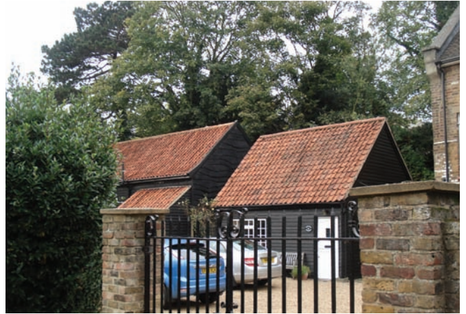
Fig.12: Notable and distinctive use of weatherboarding and clay pantiles to these vernacular buildings which make up the group of outbuildings to Woodlands (now demolished)
