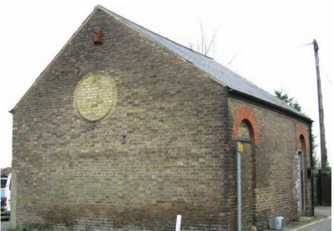
Fig 29. Former Pump House, Bell Lane.
