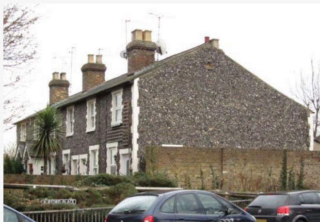
Burford Place, terrace built in 1872. The use of knapped flints is striking, a regionally distinctive technique.
