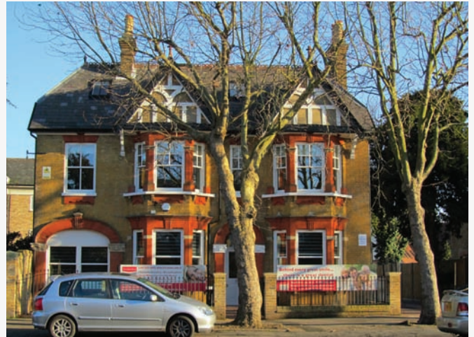
Dental Practice, High Street, opposite The Grange. Skilful use of the inherent colours of yellow and red brick and of tile, in a well designed Late Victorian former house.
