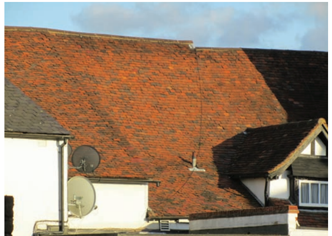
Fig.5: Handmade red clay tiles make a significant contribution to the character and appearance of the conservation area. (Rear elevation and historic ranges to the White Swan, High Street)
