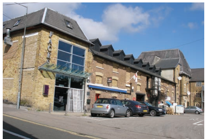
Fig 32. Former Maltings, between Brewery Road and Bell Lane.
