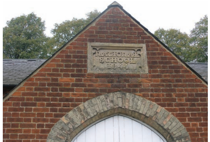
Fig 37 Red brick and Gault brick: entrance to former National School.
