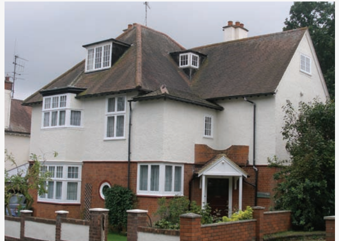
Strathavon, Yewlands. An attractively designed Arts and Crafts house of c1905 with a typically free approach to elevational design.
