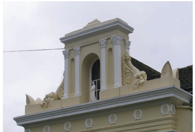
Fig.13: Stucco detailing and dressings are seen to some of the classically inspired buildings to this part of the conservation area (former stables to Woodlands, Woodland Close)
