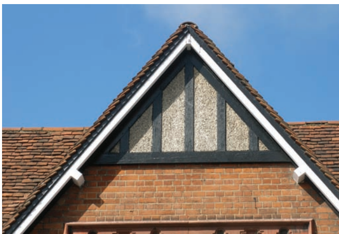
Fig 39 Red brick, plain tiles, terracotta timber framing. Roughcast and terracotta. 'Swagga' High Street
