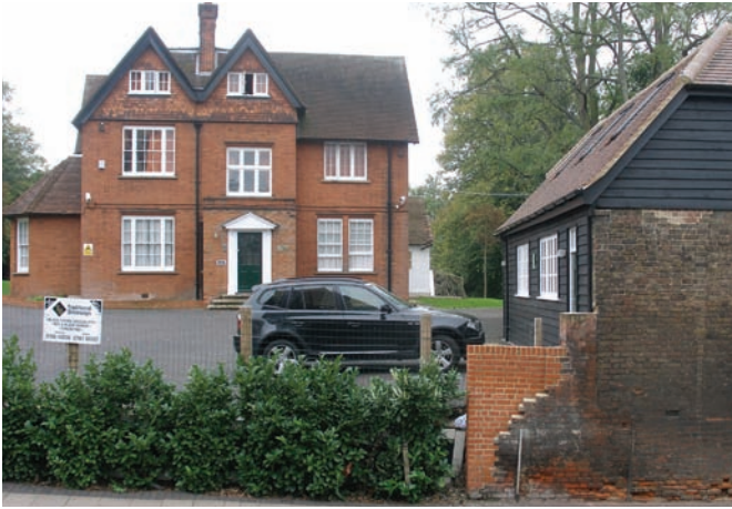
Fig 27. House and outbuilding, north side of Parish Church, Amwell Street.
