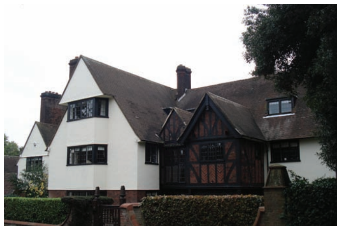
Fig.18: Yewlands (1909) by Geoffrey Lucas (Grade II listed). An extremely well-detailed house reflecting the local traditions of timber-framing, plaster and also including the architectural trademark of Lucas, the projecting gable over canted bay.
