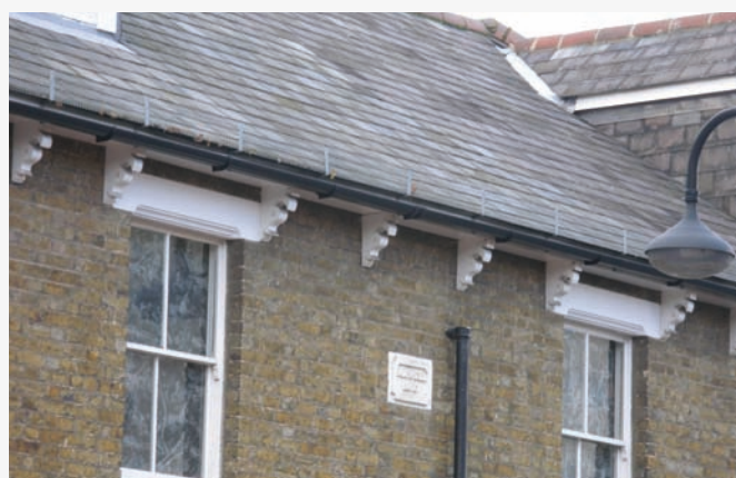
Amwell Terrace, detail of eaves brackets, original windows and plaque
