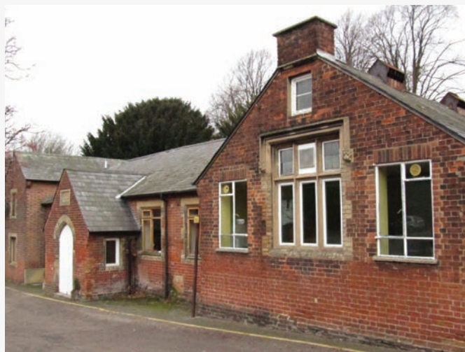
Barclay Hall, former Boys National School fronting onto Paul's Lane.
