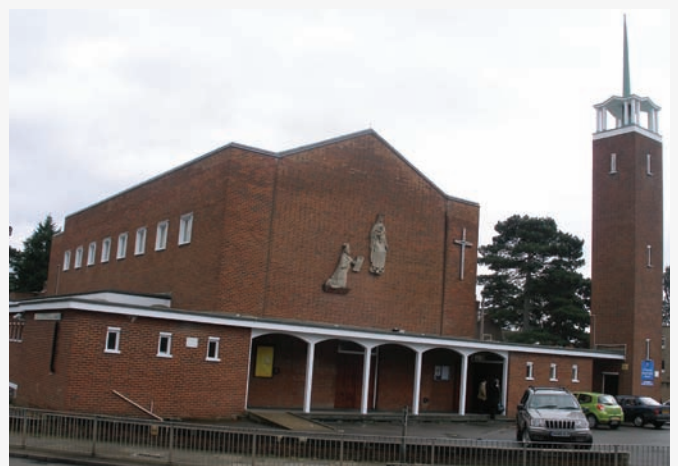
St Augustine's Roman Catholic Church, a good example of an early post war church, with an exceptionally fine landmark tower.
