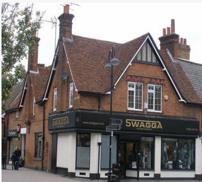
Former Three Cups Coffee Tavern facing the High Street and Lord Street.
