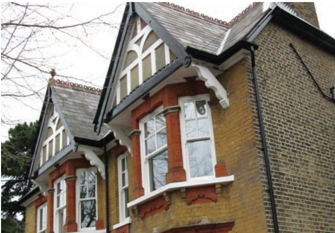
Fig.11: Dental Practice, High Street. c1897. Good use of contrasting brick colours for window and door dressings.
