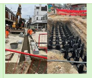
Park Lane to northern end of the High Street (adjacent to Wickes) Excavation for tree cell installation, backfilling of diverted electricity cable, excavation for kerb braces, parking bays and footpath concrete foundations.
