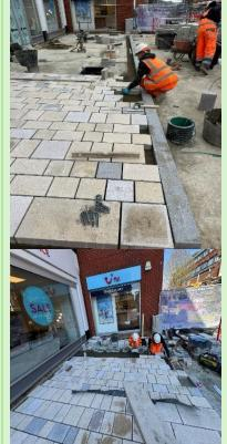
Park Lane to northern end of the High Street (adjacent to Wickes) Continued drainage works and excavation for kerb braces, new road alignment, parking bays and footpath concrete foundations.
