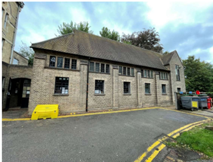
Figure 17: A view of the external walls
