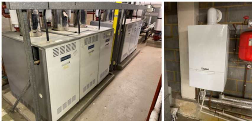
Figure 19: Floor standing gas boilers (left) and wall hung gas boiler (right)
