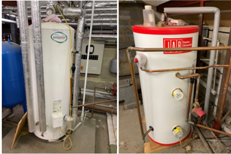
Figure 20: Electric calorifiers
