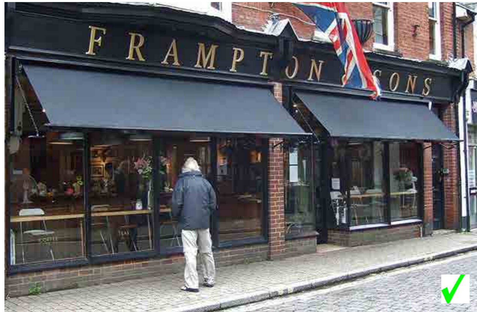
This is a good example of canopies that have been designed to fit within the framework of the shopfront and have colours that are sympathetic to the building.
