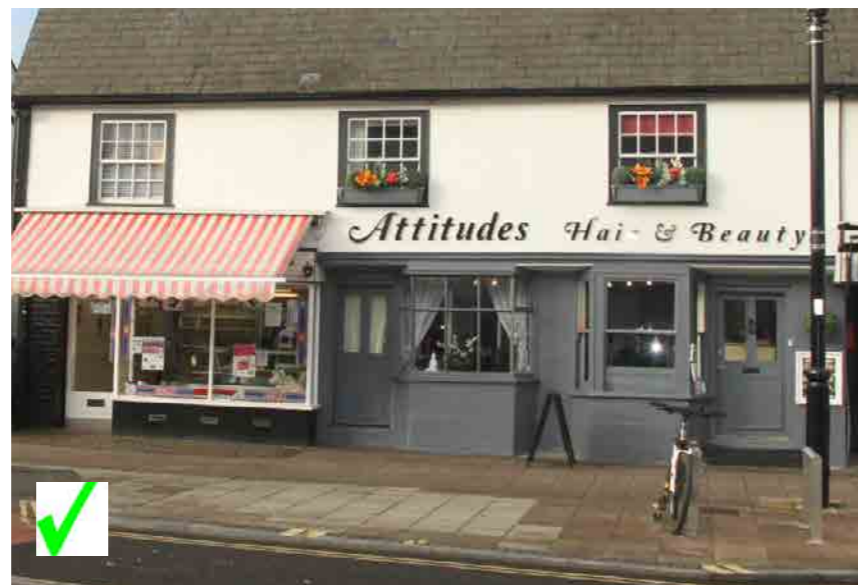
The shopfront on the ground floor has been designed and detailed to complement the streetscape
