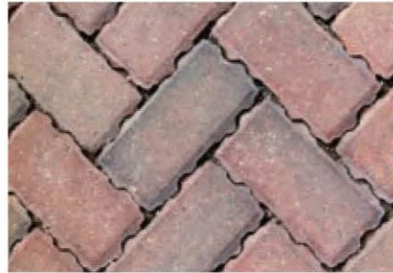
Permeable block paving with gaps in edges to allow water to soak through
