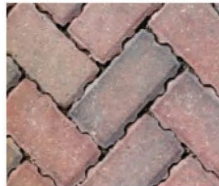
Permeable block paving
