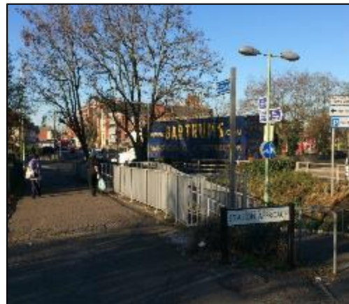
Guard railing and confusing signage
