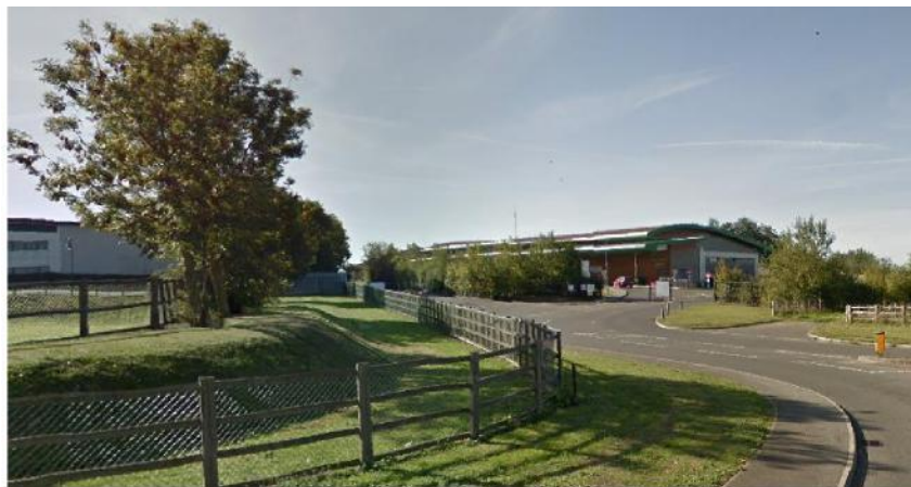
Figure 3. The Witchford centre's low-profile green roof. Image Google Earth
