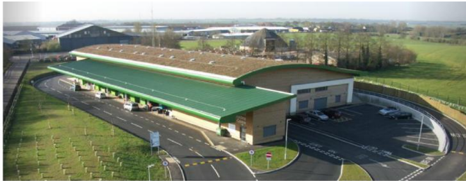
Figure 2. The Witchford centre incorporates wood cladding and a living green roof. Image: soprema.co.uk
