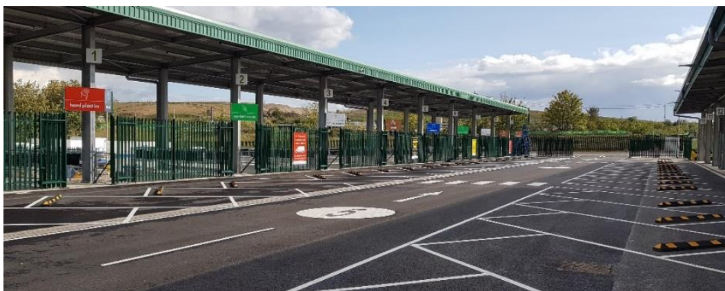
Figure 10: Ware RC supersite facility.
