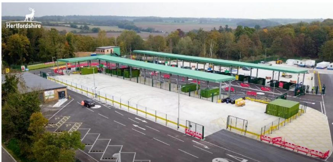
Figure 1. The Ware Recycling Centre.
