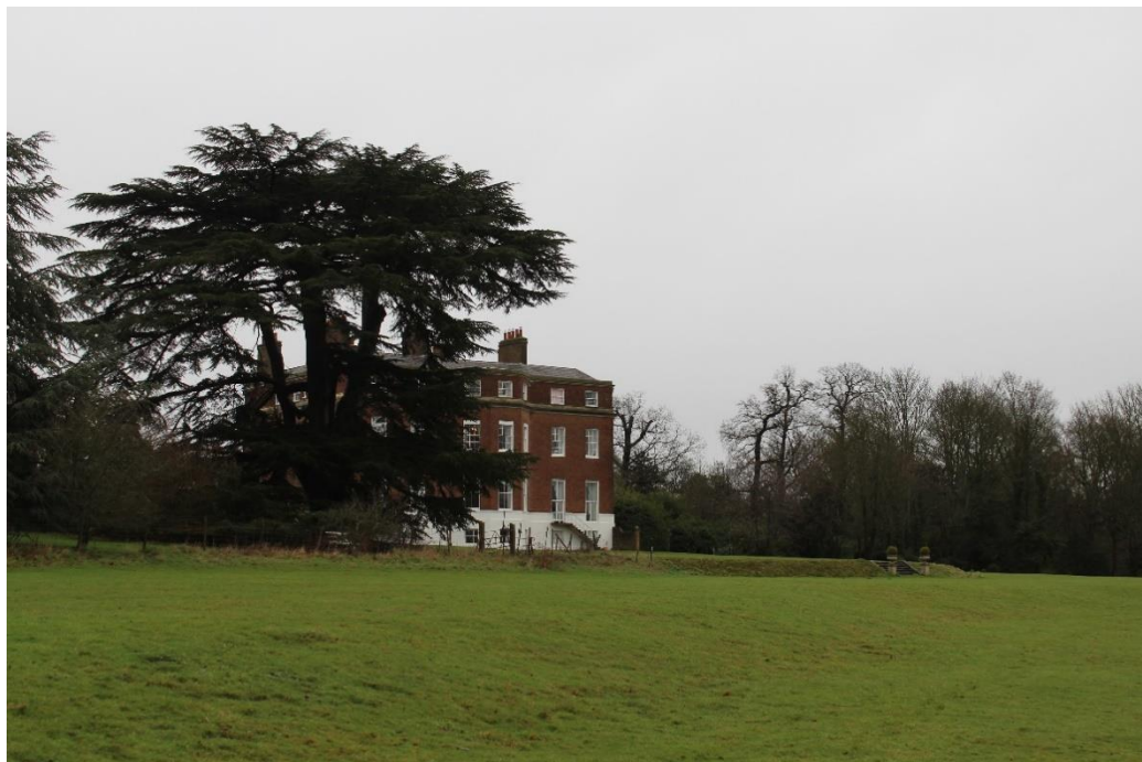
Figure 17: Wormleybury house within the registered park and garden
