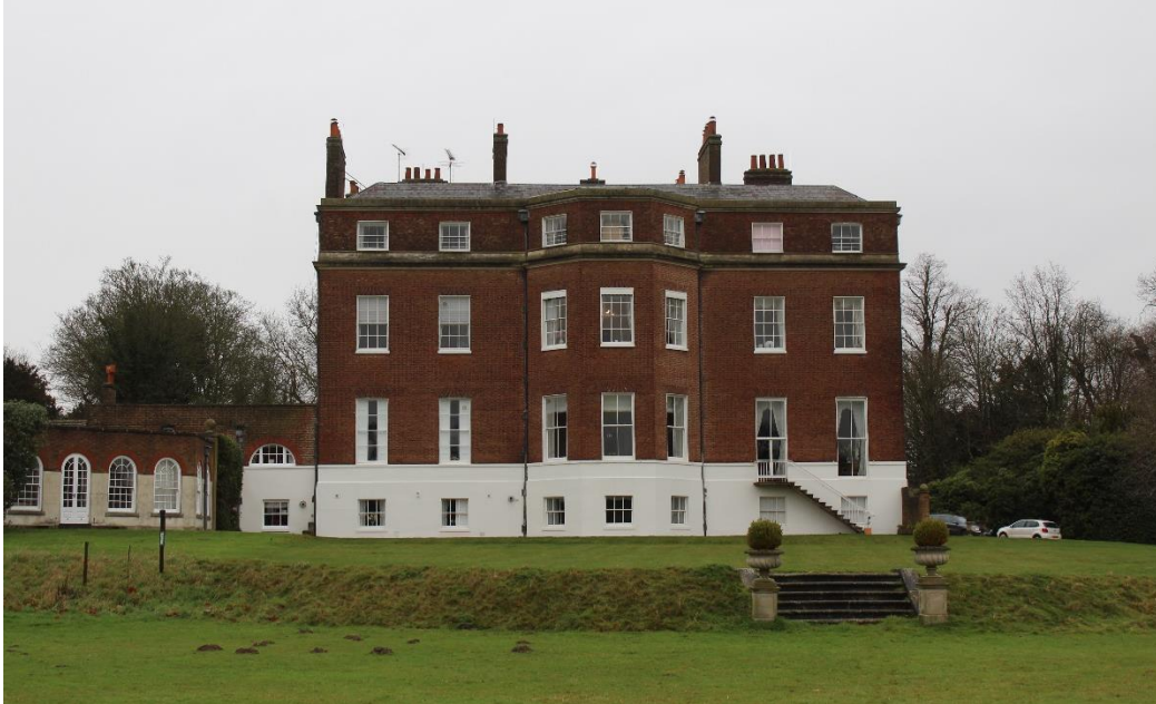
Figure 18: Rear (garden) elevation of Wormleybury house
