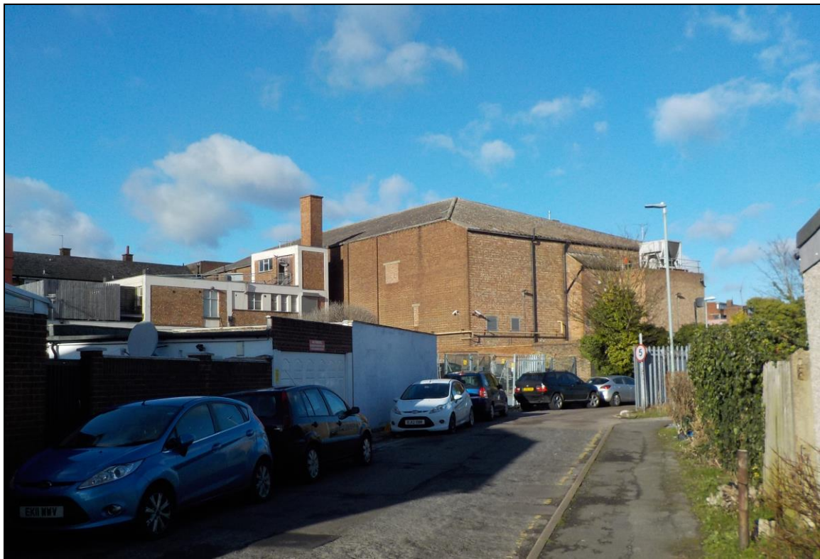
Existing rear of building and service road
