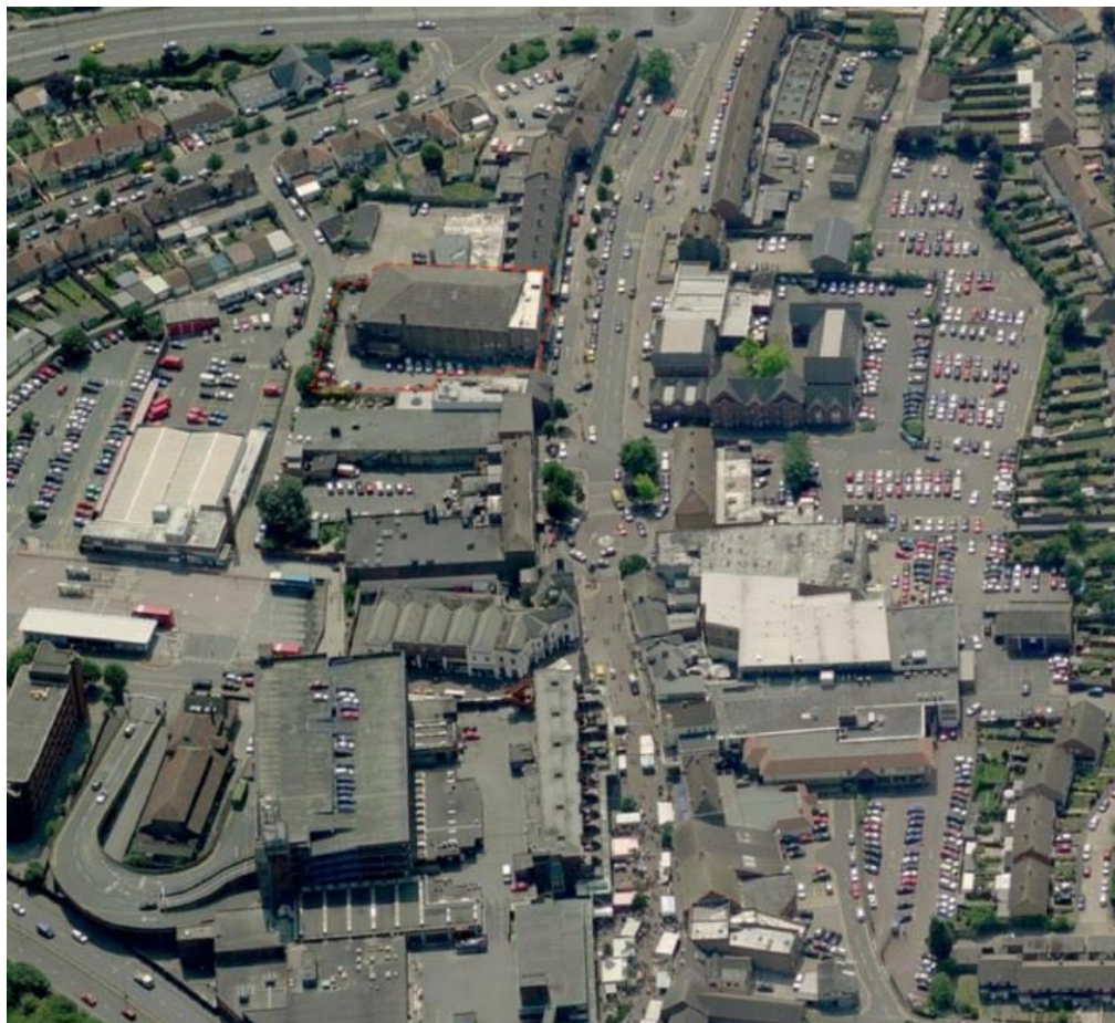
Aerial photo of the application site
