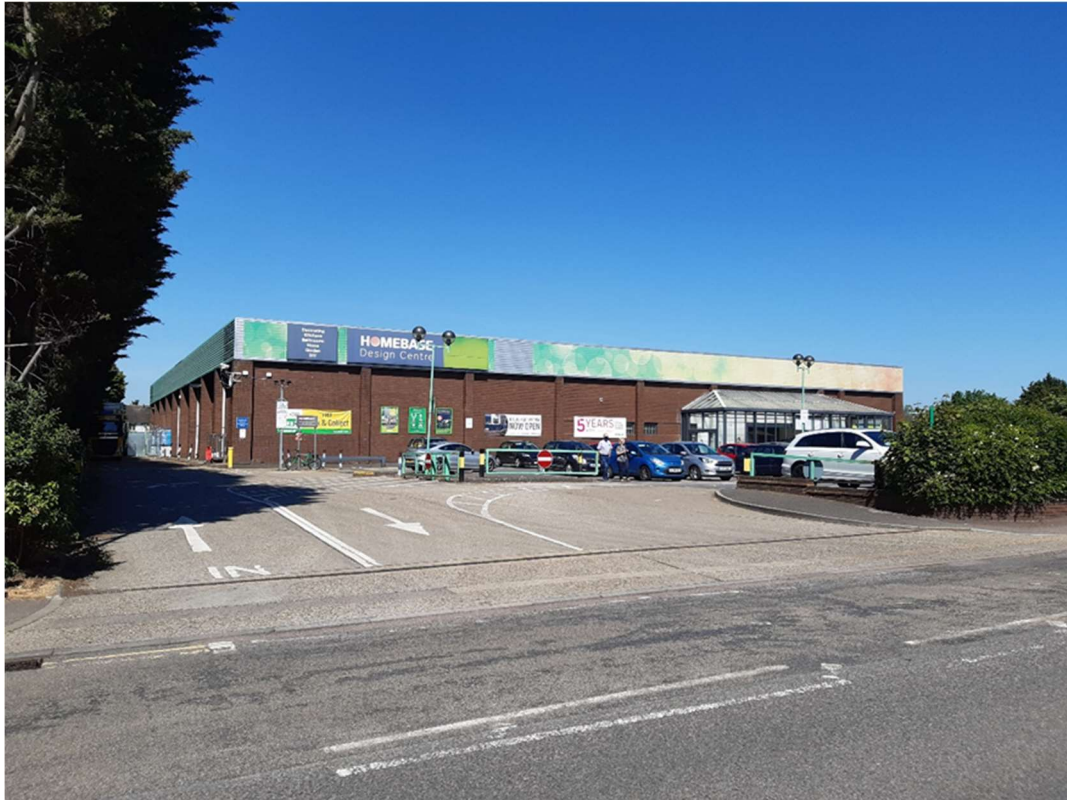
Site vehicular entrance and exit along Sturlas Way and Homebase east elevation
