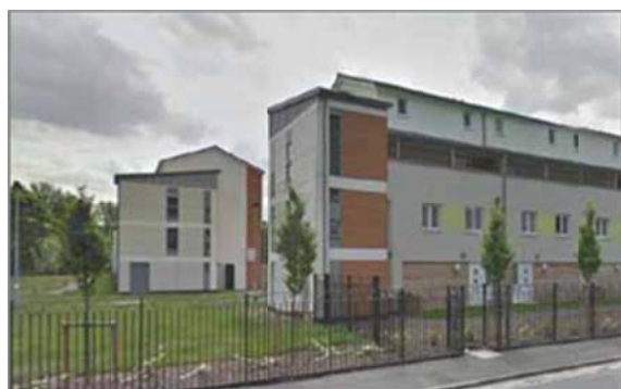
Fishers Court, Station Road– investment from B3 living has transformed the quality of this housing on a key approach to the town centre, opposite the Lee Valley White Water Centre
