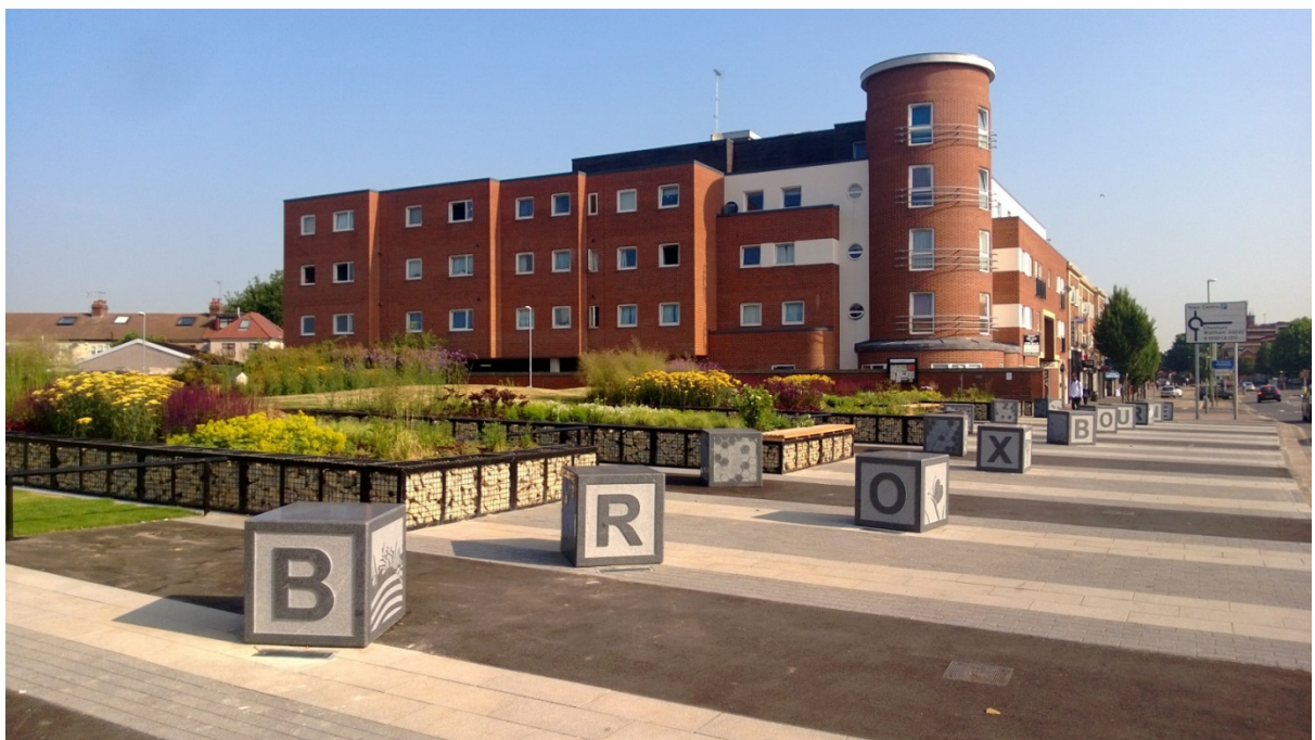
Holmesdale Tunnel open space with artwork showing Broxbourne-Enfield border
