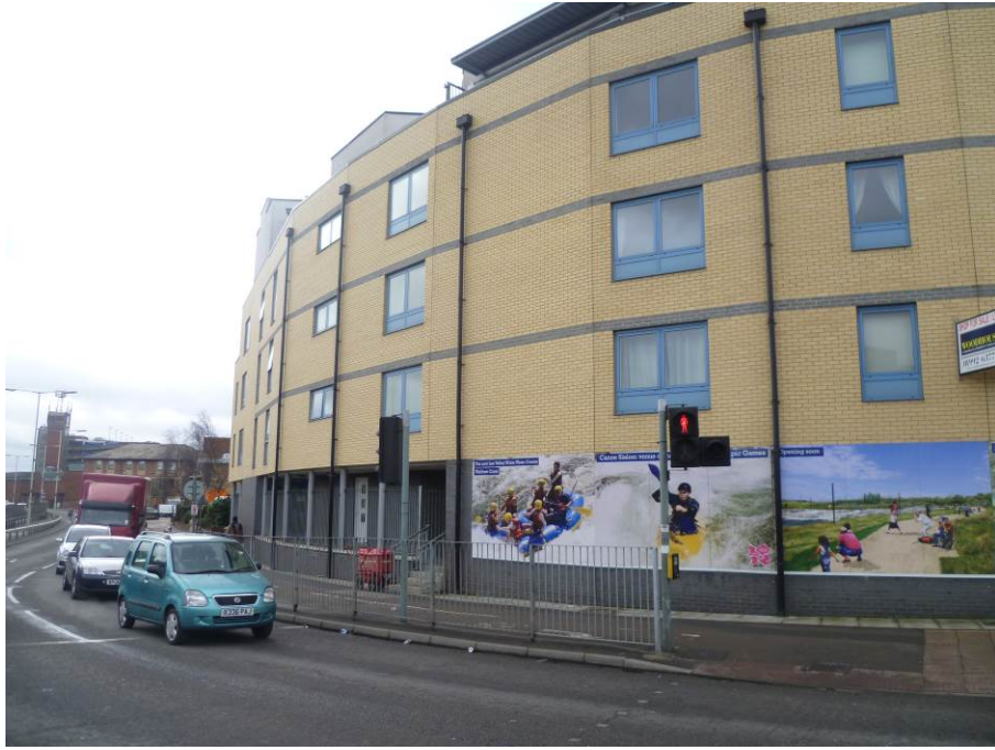
Sawyers Court, at the northern end of the High Street
