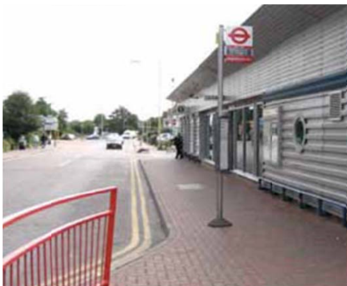
Eleanor Cross Road current public realm at the bus station frontage
