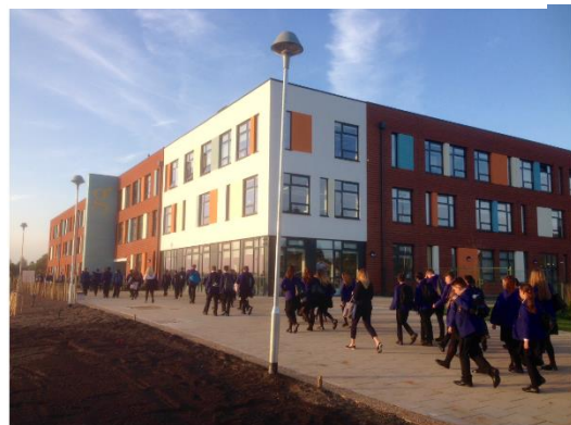
(Below) Newly rebuilt Goffs School, October 2017
