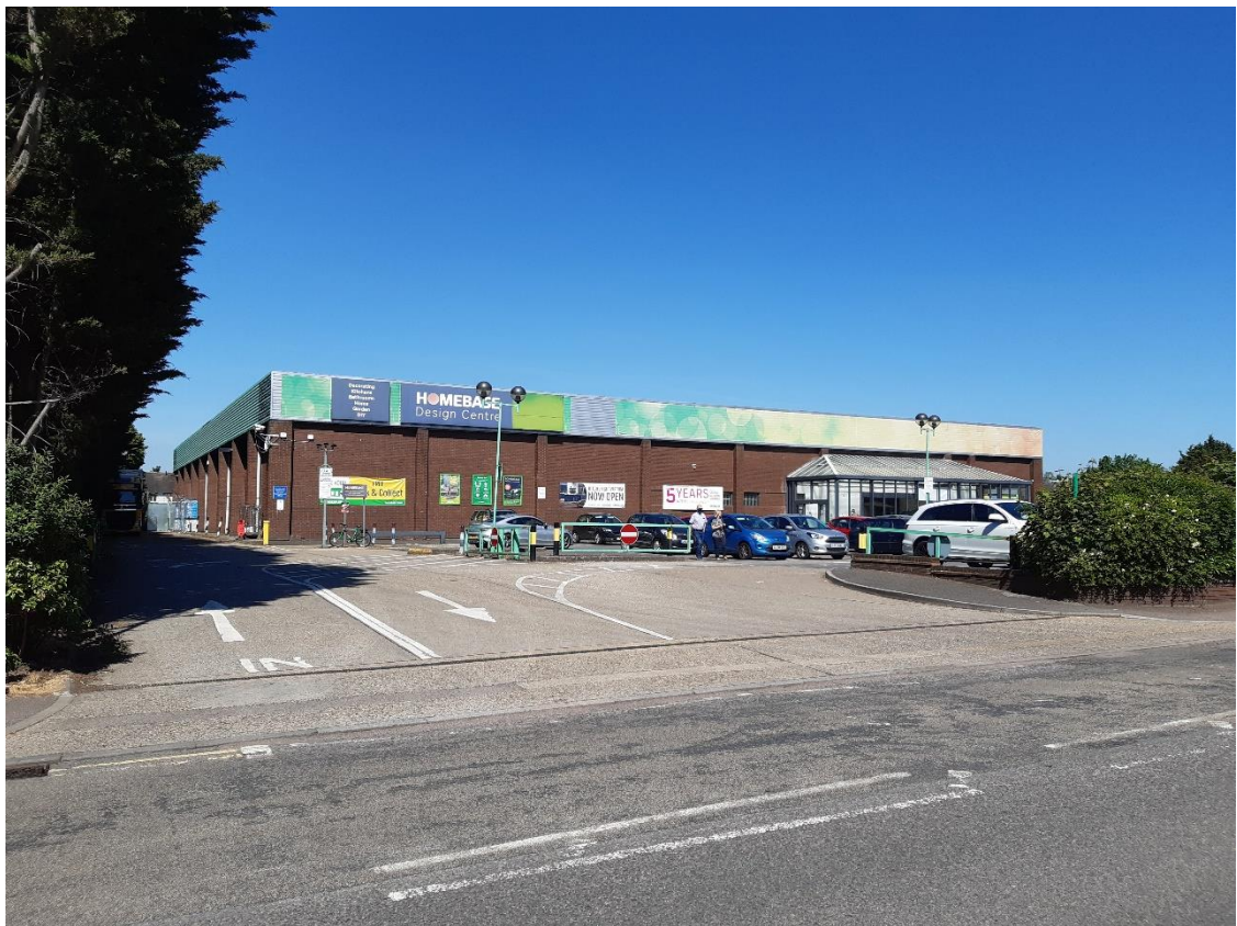
Entrance, east elevation and southern service area
