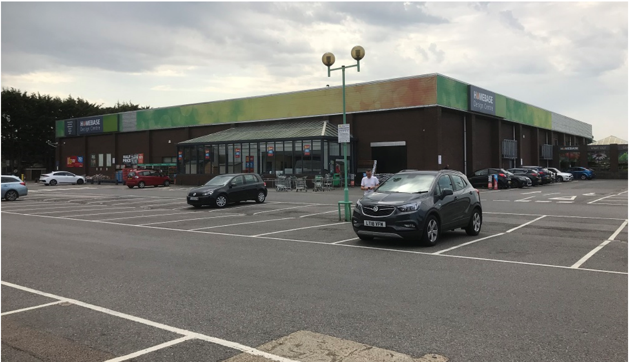
The car parking around the front and side of the Homebase Unit.
