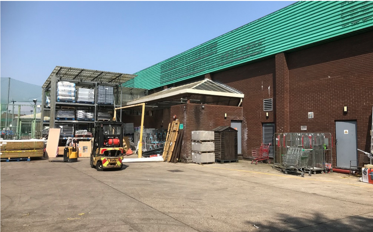
Storage area at the rear of the Homebase Unit.
