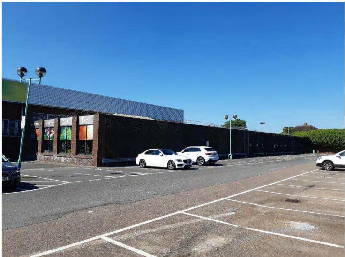
North elevation (Garden centre structures proposed to be demolished)
