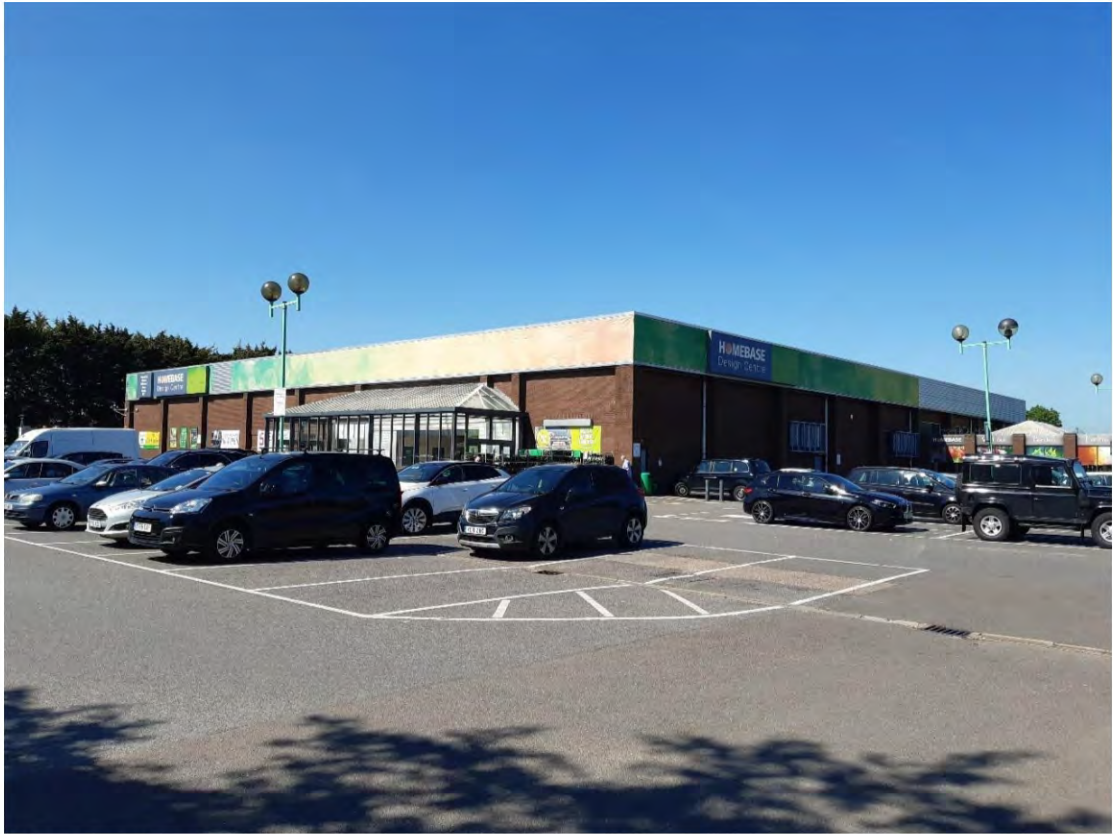
North east corner of existing Homebase store
