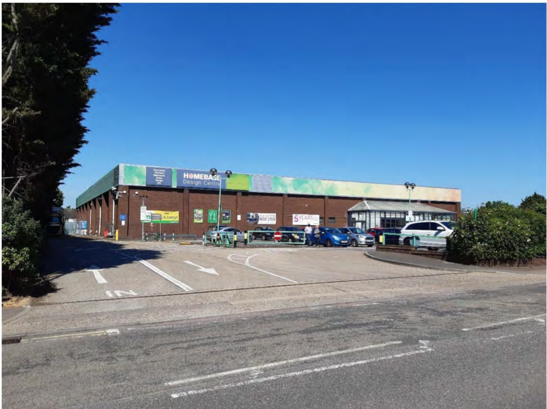
Entrance, east elevation and southern service area
