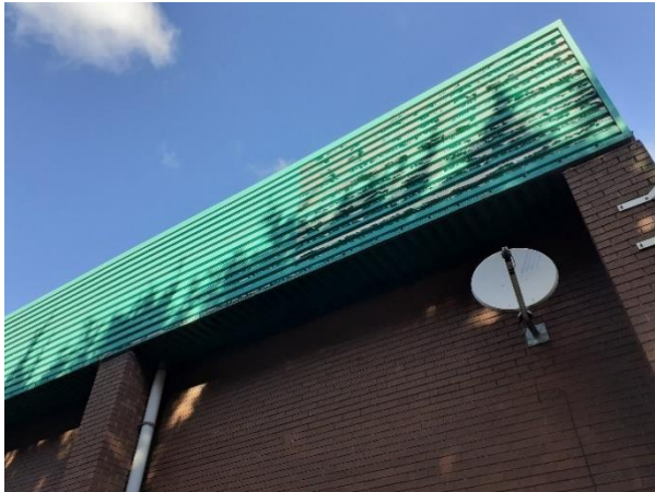
Photograph 3.5 View of the exterior of building B1
