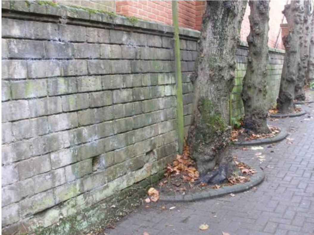
Wall constructed in patent Hitch bricks
