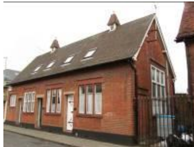
Former Temperance Hall; with carved neo Tudor lintels and ridgeline roof vents.
