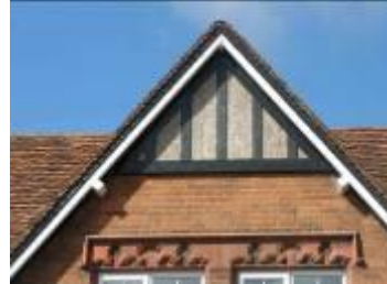
Detail of gable and lintel
