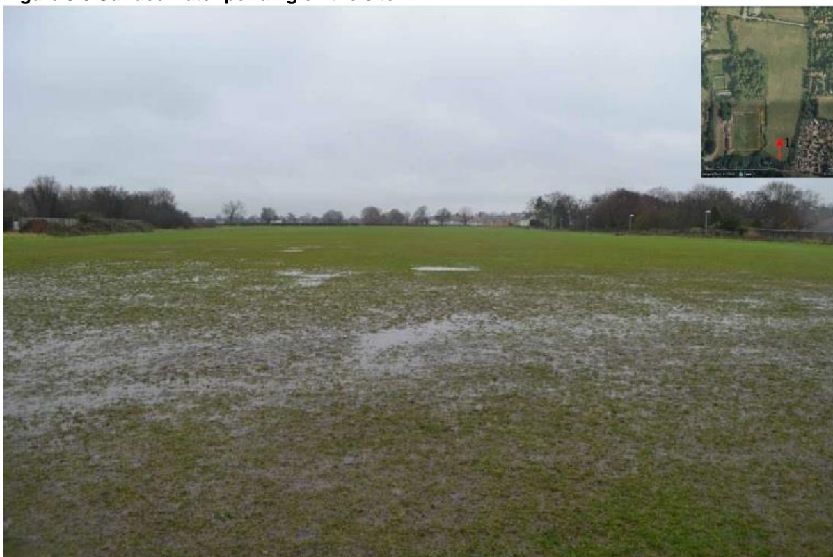
Figure 3-9 Surface water ponding on the site
