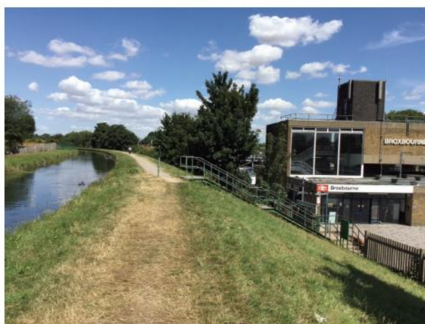
Broxbourne Station and the New River
