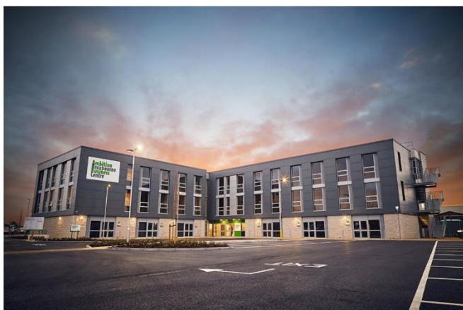
(Below) Ambition Broxbourne Business Centre
